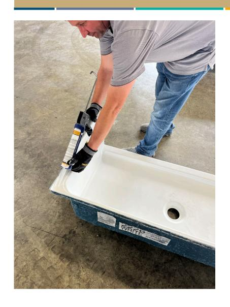
Apply a 1/4" bead of silicone caulk around the top of flange.
