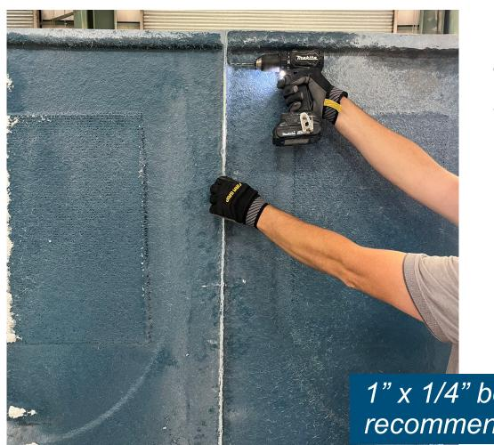
Pre-drill holes on the back panel vertical flange, 12" apart.
