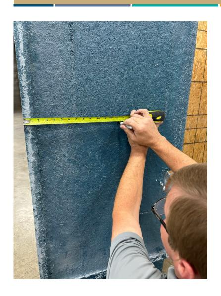
Mark holes needed for plumbing fixtures on back of unit.
